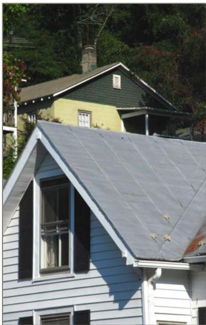
**Gable:** the triangular wall segment at each end of a double-pitch roof, often referred to as a gable roof.
