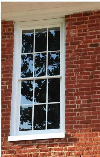
**Light:** pane. Individual glass-covered opening in a window. Often used with reference to the number of panes in a window sash, such as “6 over 6” or “9 over 9.”
