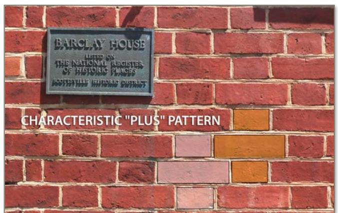
▲ **Flemish Bond:** brick bonding characterized by using alternating headers and stretchers in each course or row.
