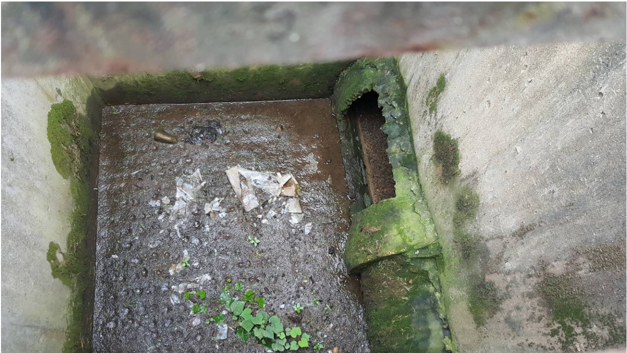
Image 2. Drainpipe within drainage inlet structure.
