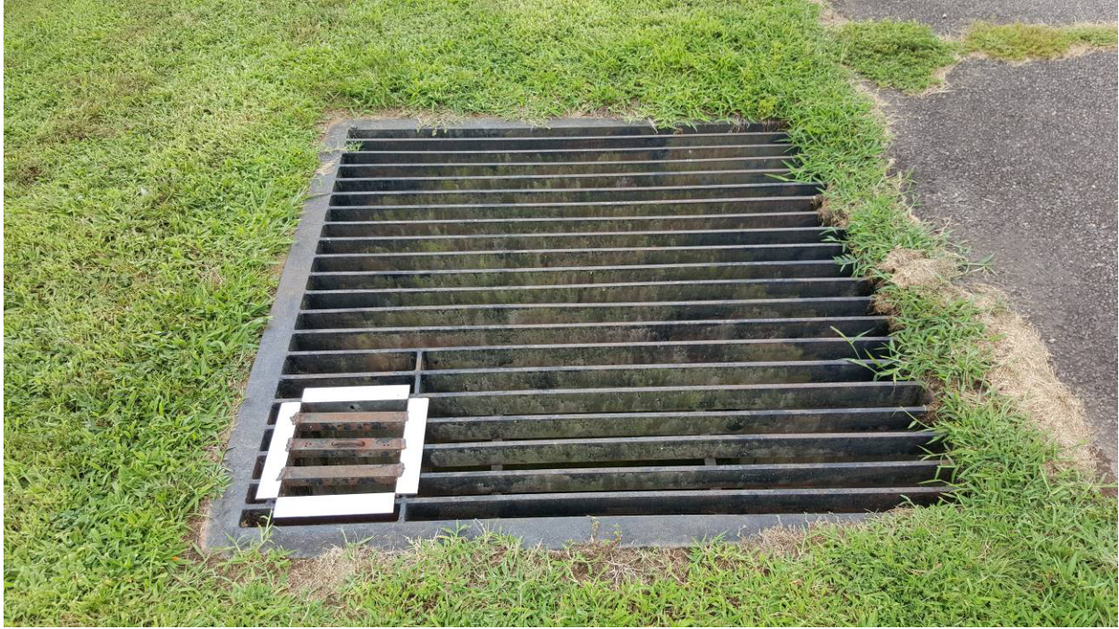
Image 4. Drainage inlet with access hatch for portable pump suction line.
